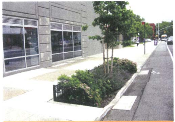
Bioswales use planted areas to reduce drainage
