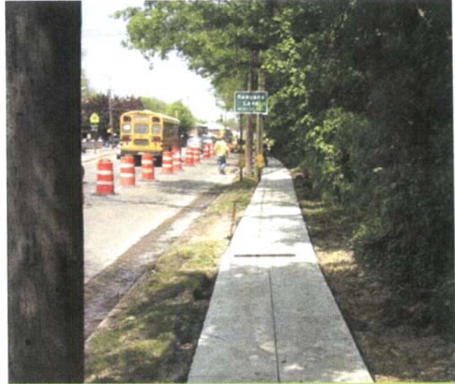
After: Hylan Boulevard—Rubber sidewalk, trees saved
