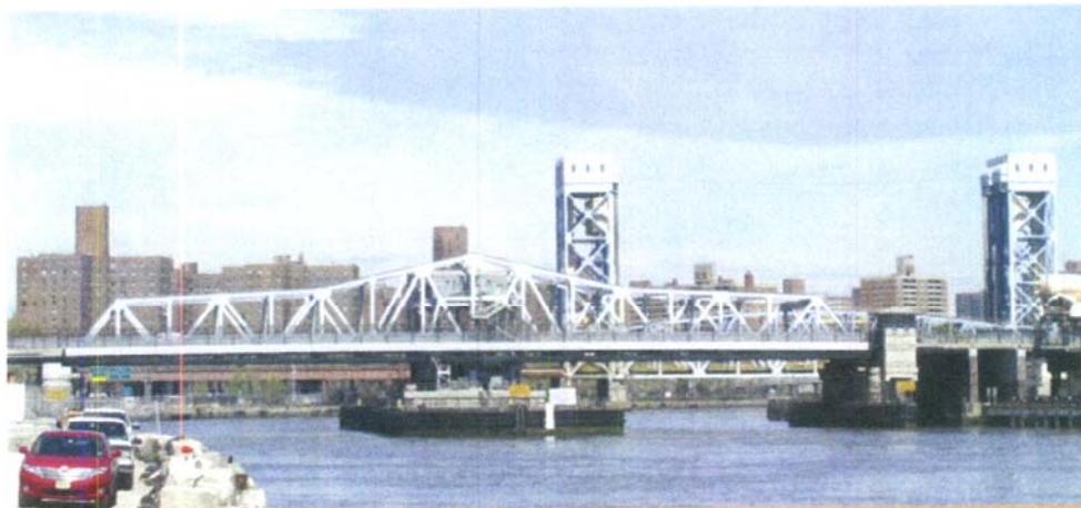
3rd Avenue Bridge
