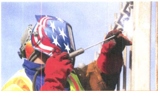
DOT worker fixing Brooklyn Bridge
