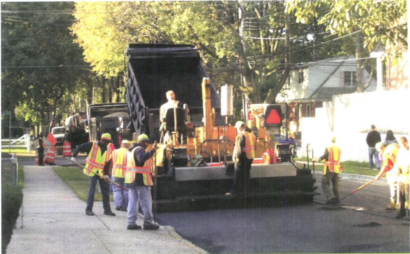
Warm mix asphalt being laid in Queens
