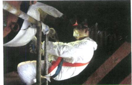
Installing strain gauges on a movable bridge – Pulaski Bridge over Newtown Creek
