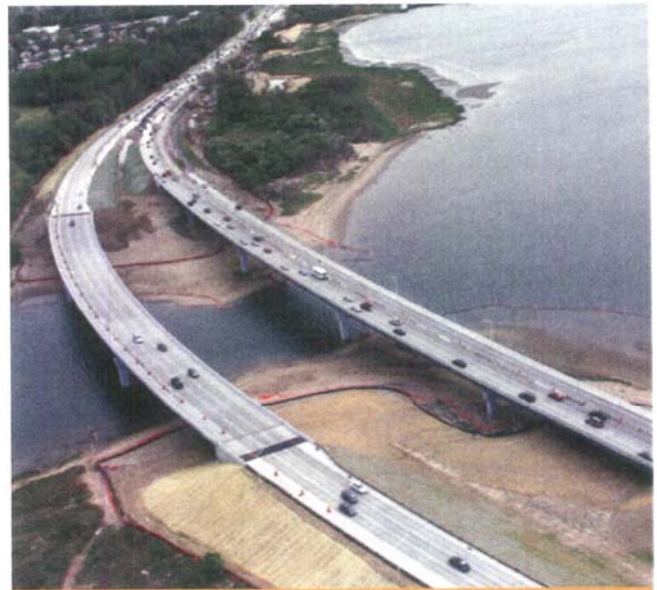
New Paerdegat Basin Bridge in Canarsie.
