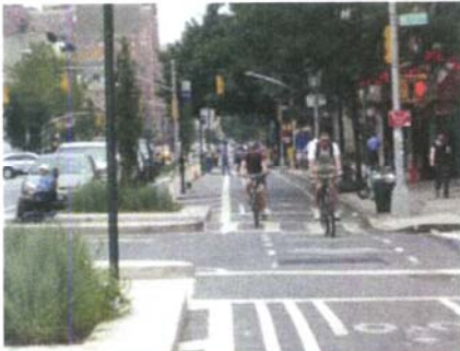
Counts have shown a 57% increase in the number of cyclists using 9th Avenue since installation of the parking protected bike lane
