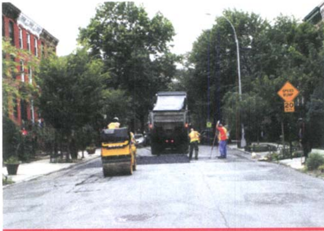
Speed bump installation
