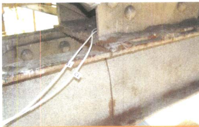
Strain gauge monitoring of beam on the Brooklyn Bridge
