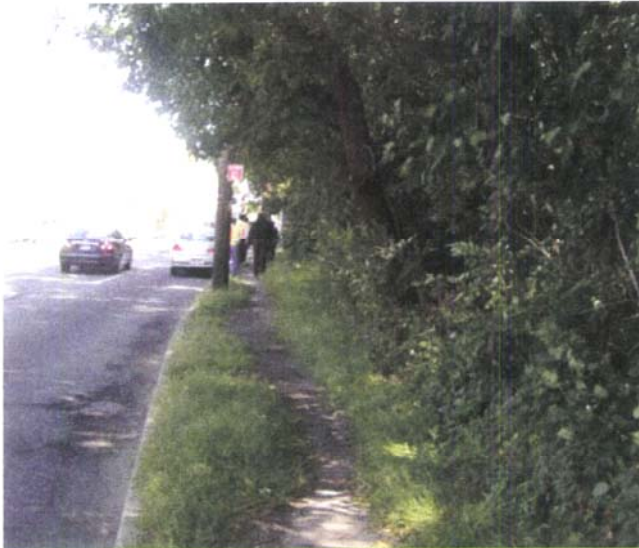
Before: Hylan Boulevard—No sidewalk
