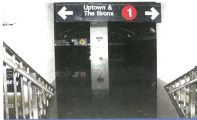
Flooding at South Ferry subway station after the storm
