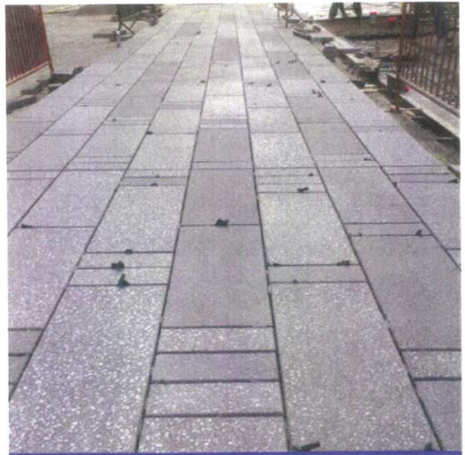
Pavers being installed as part of Times Square reconstruction project
